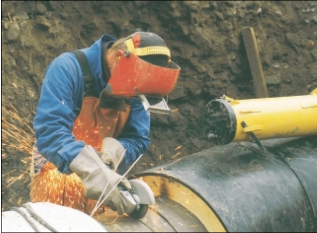
Welding in PUR insulated steel pipe.
