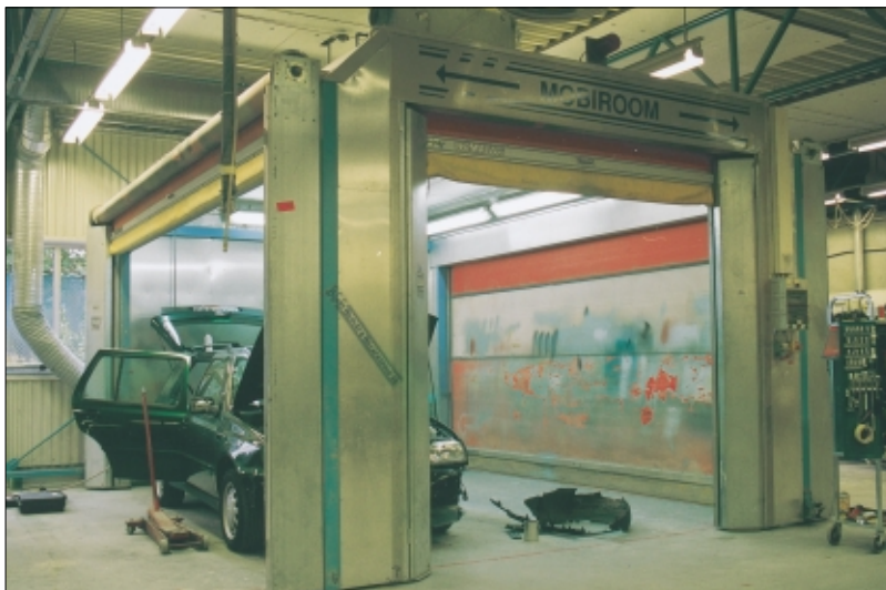
A mobile booth can be used to isolate the "isocyanates work" in the car repair shop.
